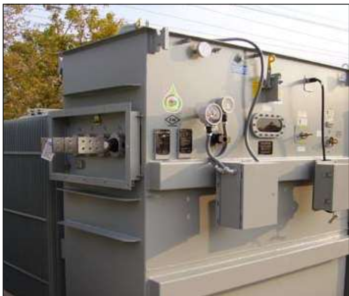
Figure 21. Substation transformer with visible break technology.
