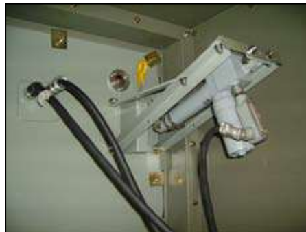
Figure 13. Motor-operator for open/close of Vacuum Fault Interrupter (VFI).
