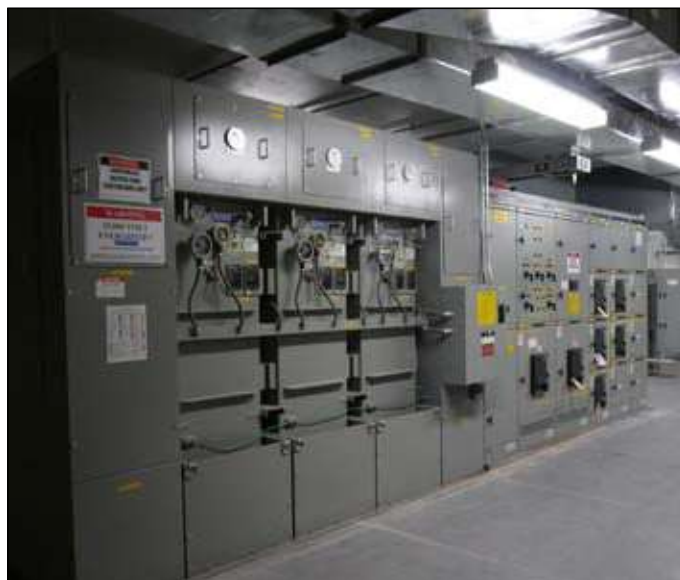
Figure 23. Triplex Indoor Power Center comprising of energy efficient and low noise single-phase substation transformers in a ganged setup.
