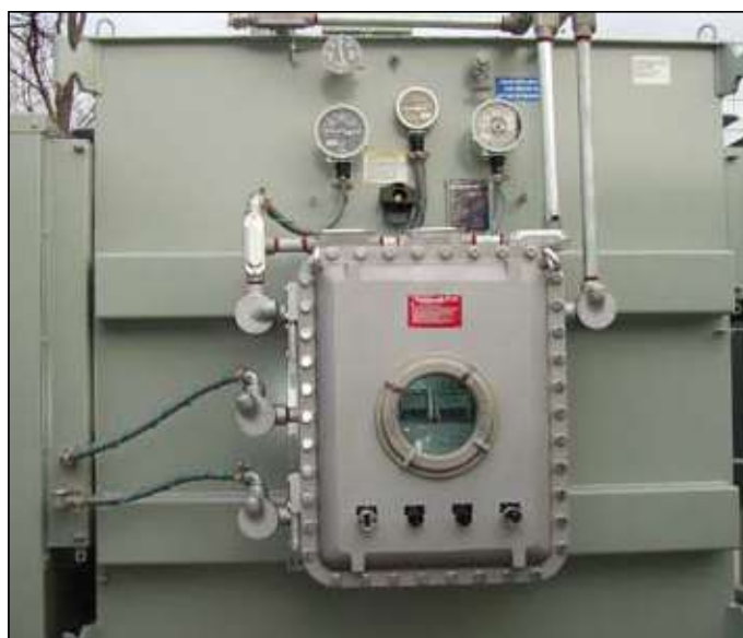
Figure 24. Class 1 Div 2 hazardous duty substation transformer.
