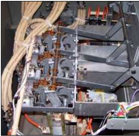
Figure 14. VFI - Inside Transformer Tank.
