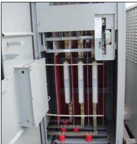
Figure 16. LIS - Interior view showing power fuses.
